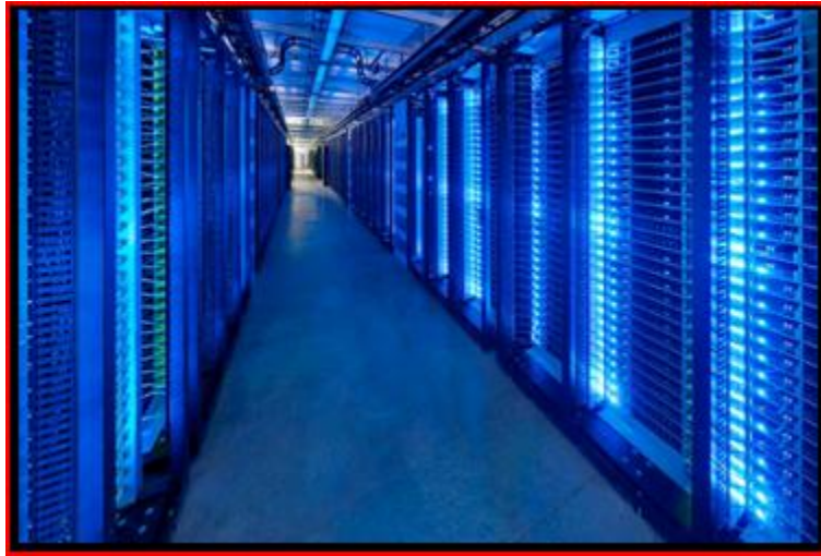
Figure 15: Servers in Data Center
